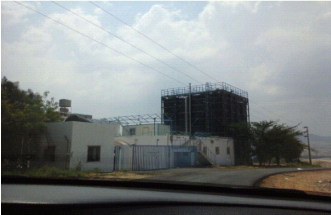
Figure (1.3-A): The Tal Mantah WWTP
