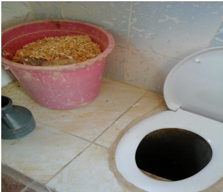
Figure (1.1-D): waterless toilet
