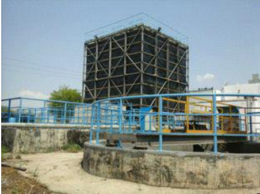
Figure (1.3-B): View of the WWTP at Tal Mantah
